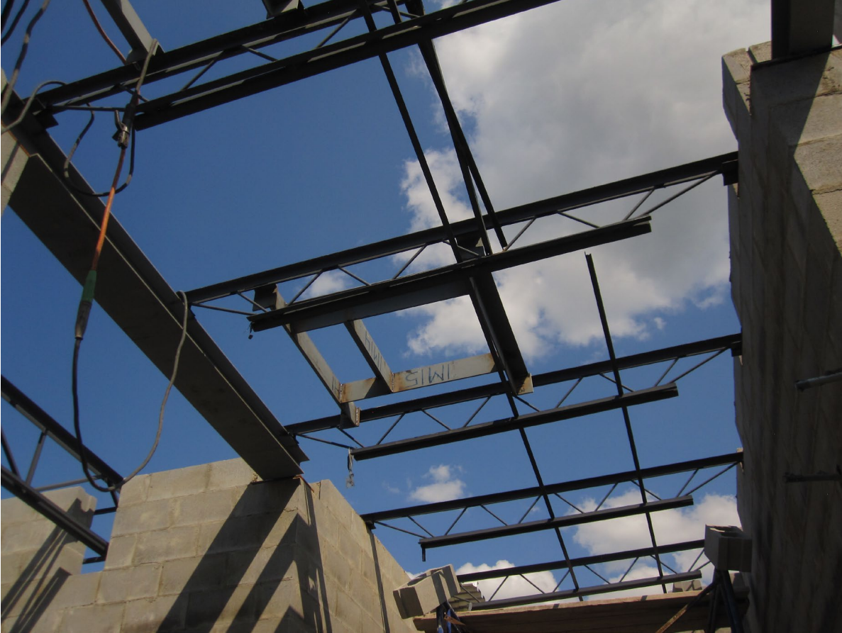
Roof of addition during construction
