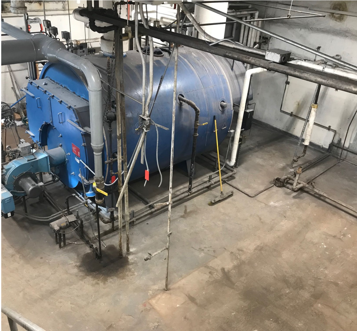
Getting boiler room ready for new boiler
