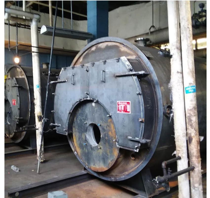
New Boiler installation in progress
