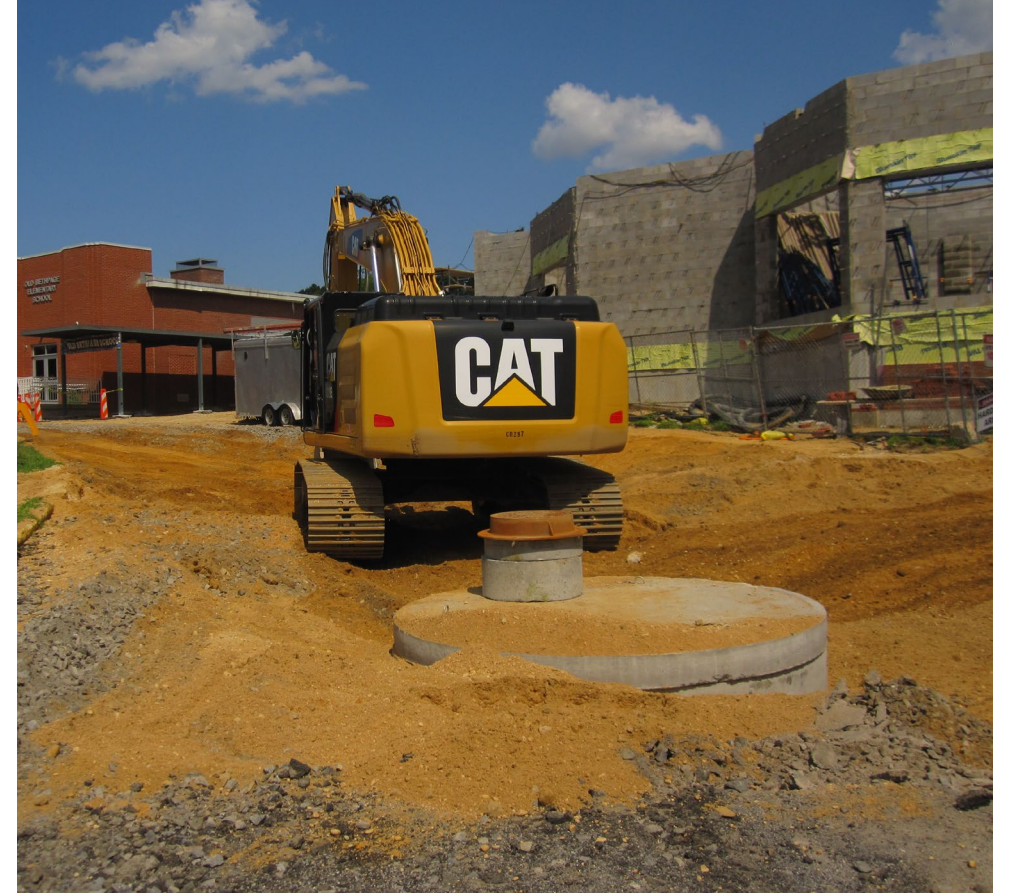
New driveway and side of addition
