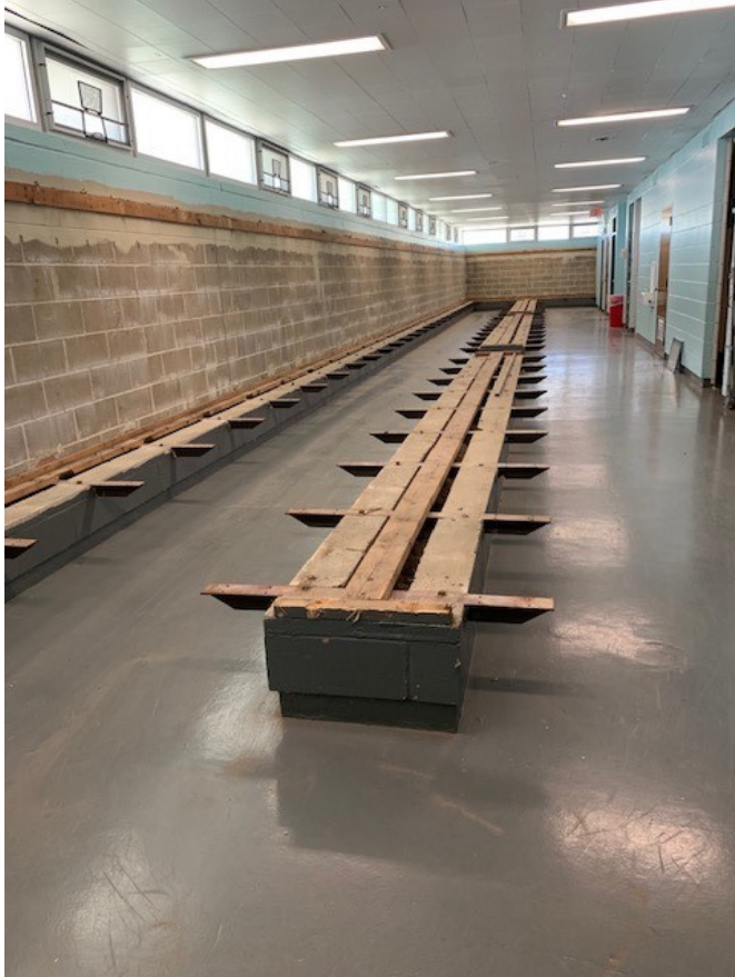
Locker Room renovation
