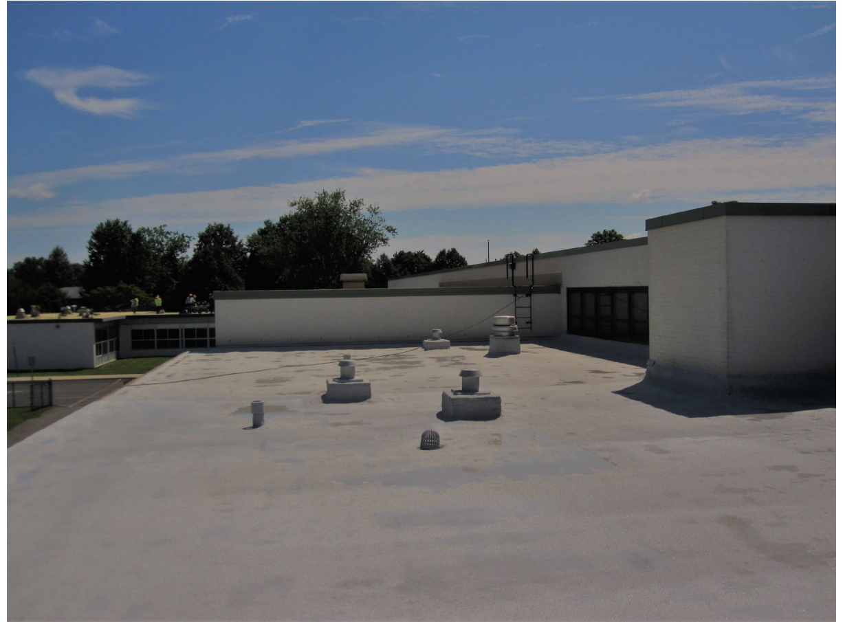
New roofing with in-house fans installed and sealed
