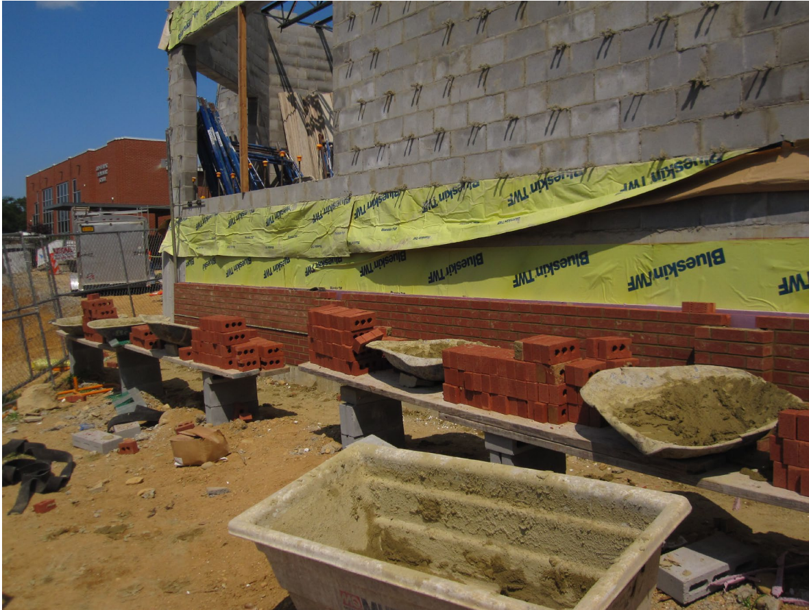
Exterior wall of classroom addition with exterior brick being installed.
