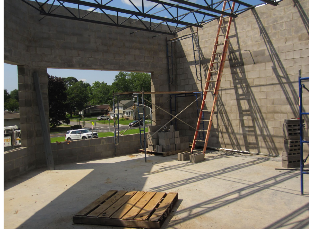
Interior of classroom addition in progress.
