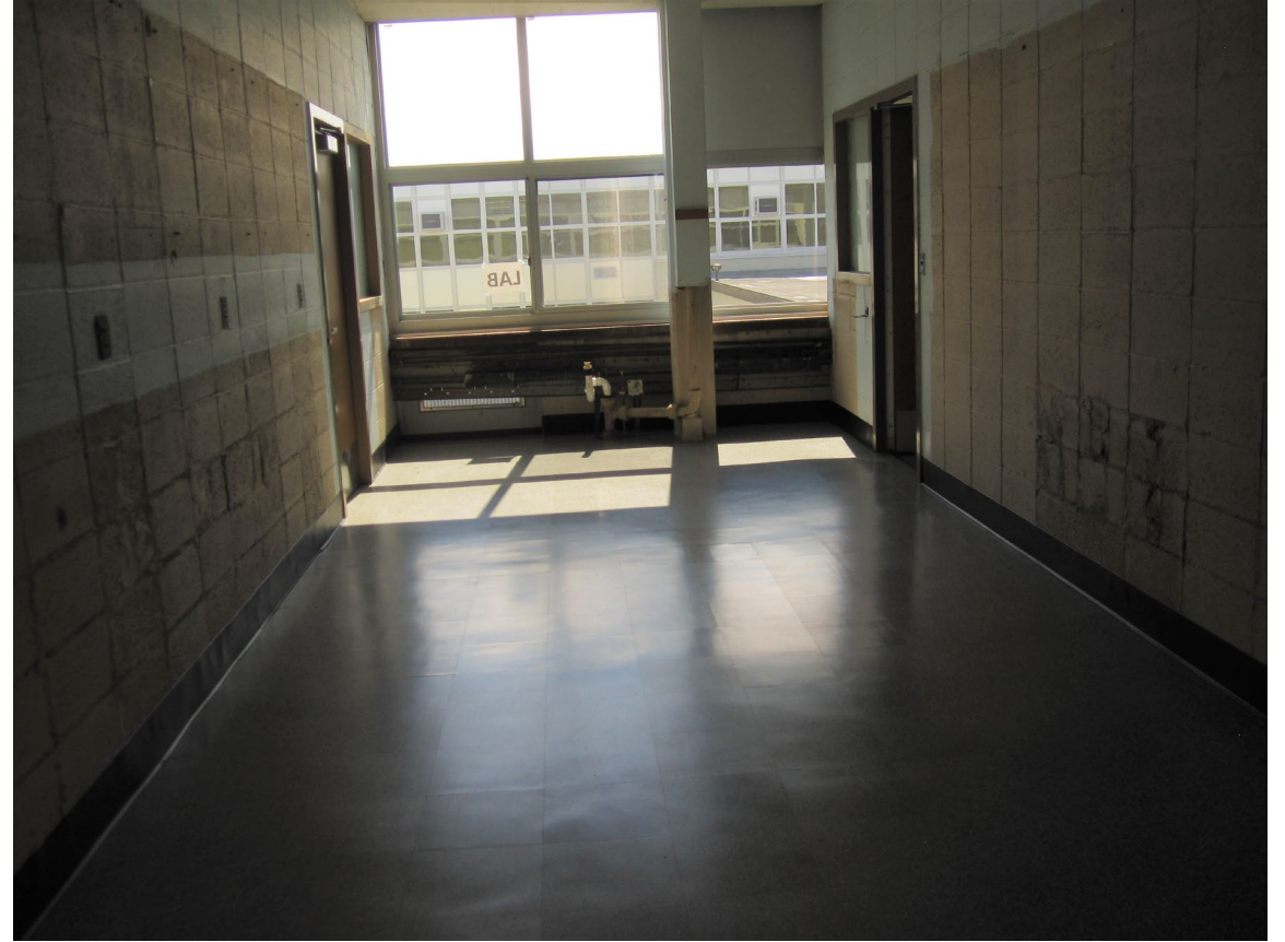
Room 302 prep room flooring installation in progress
