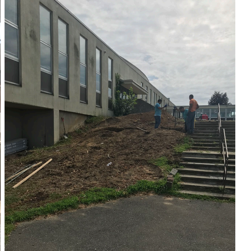
Exterior masonry retaining wall work
